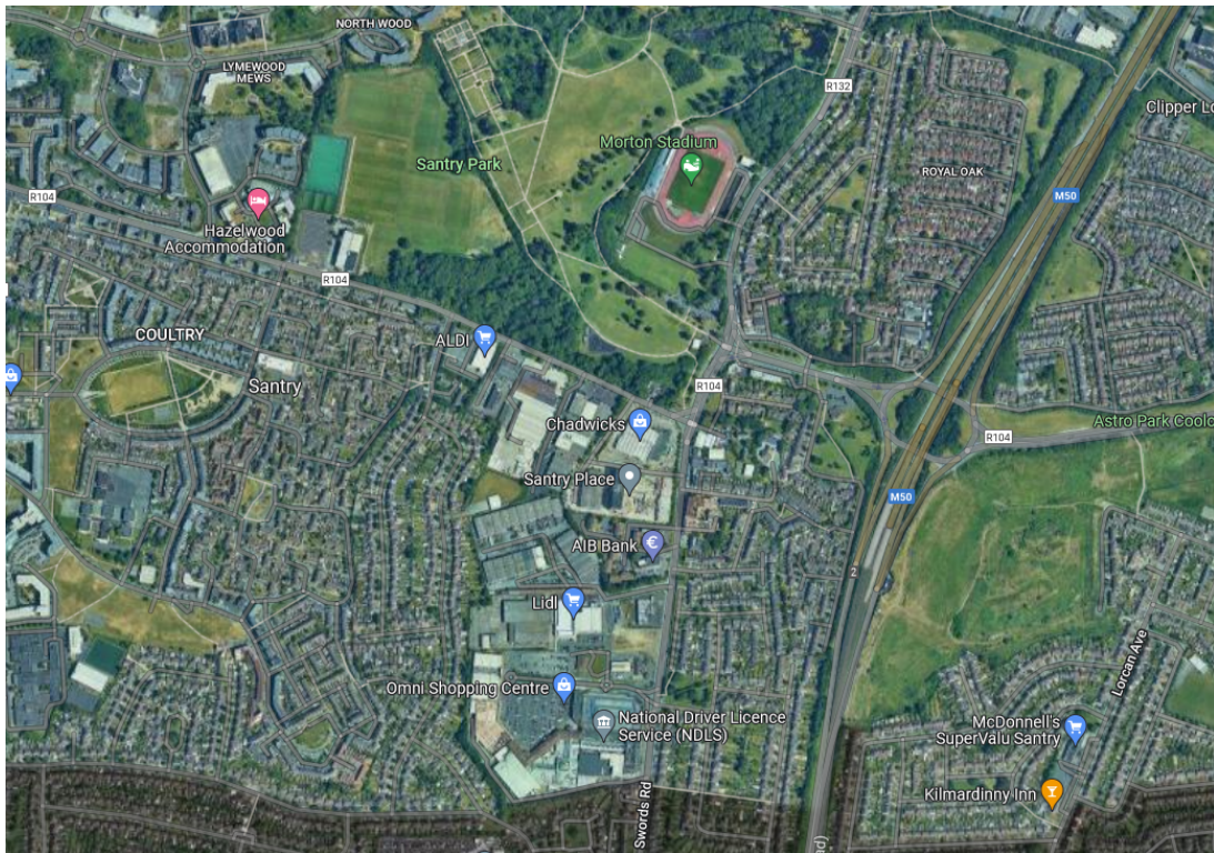
Figure 4.1: Existing Receiving Environment (Baseline Situation)
